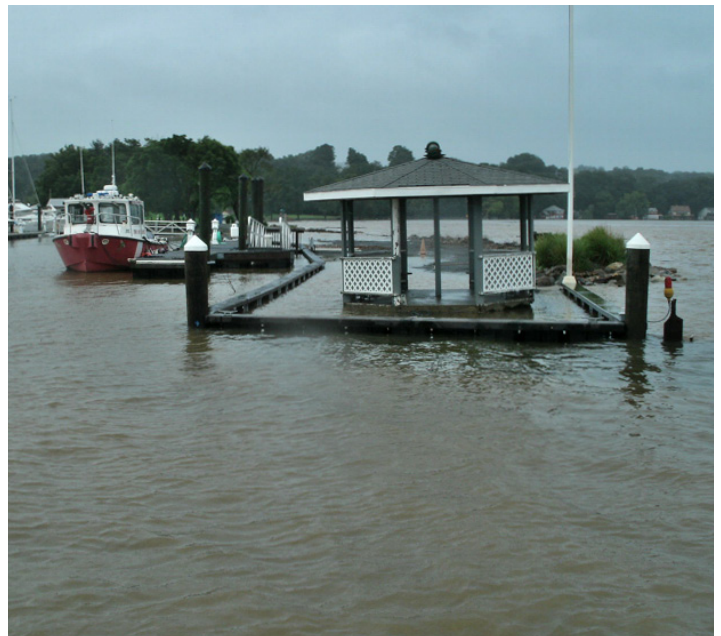
West breakwater on the morning of Sunday, August 28, during the heavy rains of Hurricane Irene and high tide. Note the extra height on the new pilings kept our boats safe.
